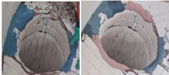
Applied mid Aug 2022 Inspected end of Mar 2023
