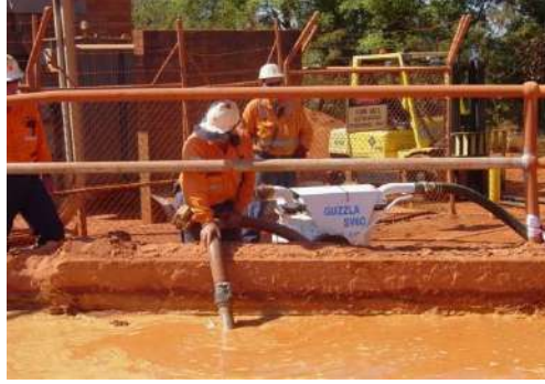
Emptying typical u/g drainage sump
