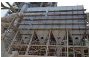
Flue gas – 200HT
