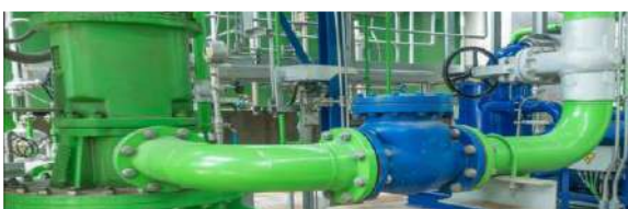
Plant wide corrosion and abrasion protection
