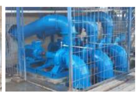
Iron ore reject tailings dewatering centrifugal pump – 356
