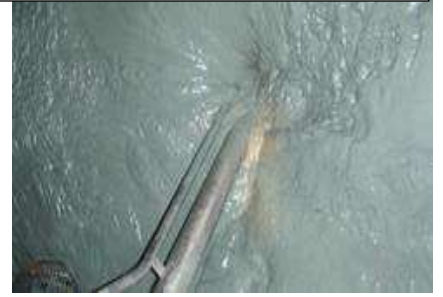
Emptying typical u/g drainage sump
