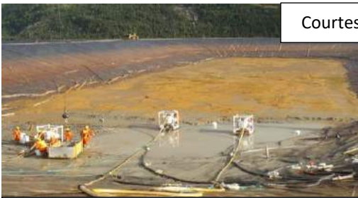
This lined mill water sludge sedimentation pond was emptied, and solids were automatically discharged 2,600 meters through three 100mm hdpe lines for disposal with zero-leaks.
