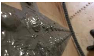
Steel tank rivet leaks – 251
