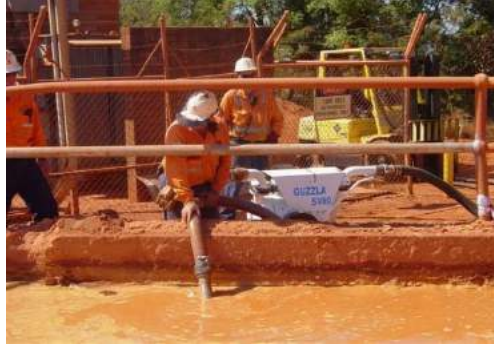
Emptying typical u/g drainage sump
