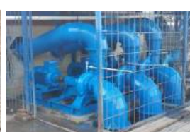
Iron ore reject tailings dewatering centrifugal pump – 356
