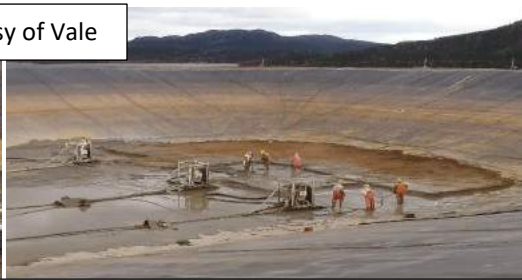
This lined mill water sludge sedimentation pond was emptied, and solids were automatically discharged 2,600 meters through three 100mm hdpe lines for disposal with zero-leaks.
