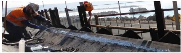
Permanently repair large belt edge & cover damage quickly w/ Melta Pro® machine. Only RubbaFIX® remains 70 durometer = will not harden & crack like polyurethane.
