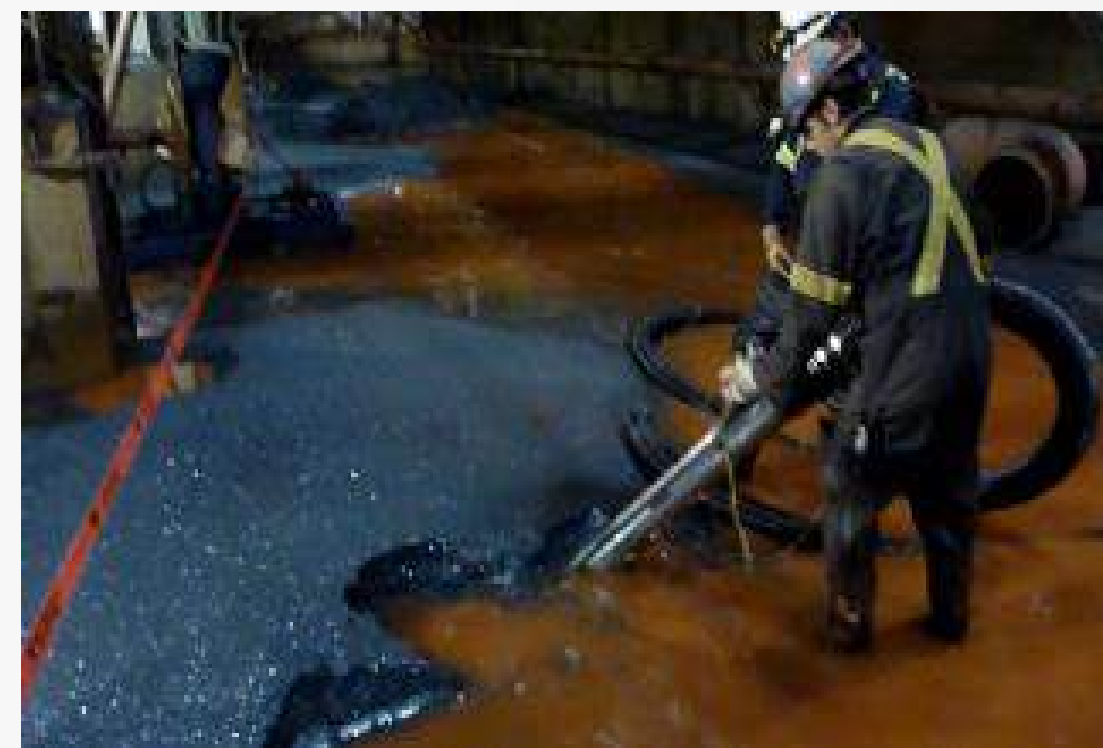
Vacuum recovery spilled iron ore concentrate.
