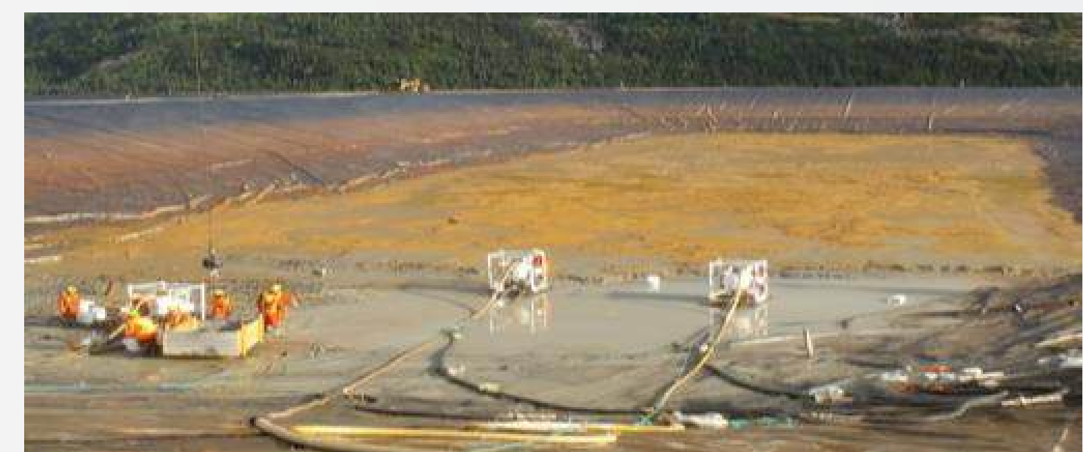
This lined mill water sludge sedimentation pond with thick abrasive solids was emptied, with solids discharged 1,390 meters (4,300 feet) through three 100mm (4") hdpe lines for disposal with no liner damage or leaks.
