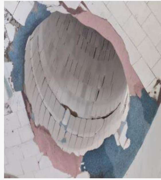
Inspected end of Mar 2023
