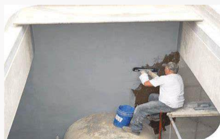
Concrete, secondary containment, flooring – 800, 830, 600, 870
