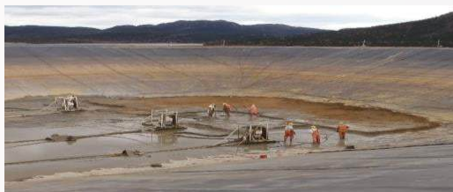
This lined mill water sludge sedimentation pond with thick abrasive solids was emptied, with solids discharged 1,390 meters (4,300 feet) through three 100mm (4") hdpe lines for disposal with no liner damage or leaks.
